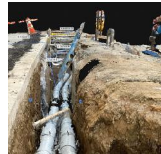
Infrastructure inspection with measurements
